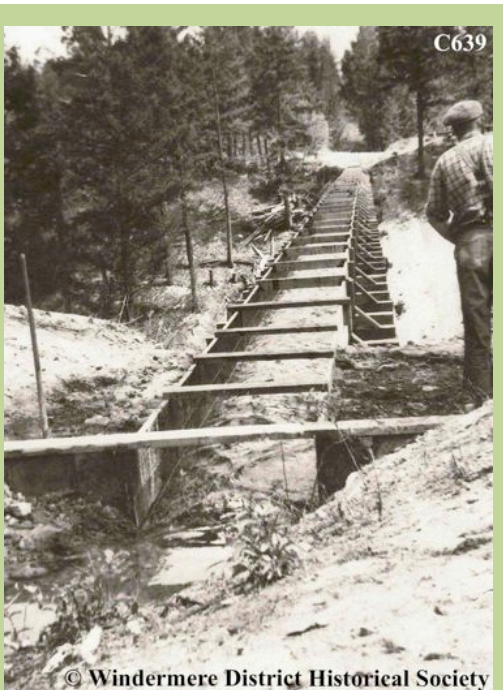
© Windermere District Historical Society Irrigation Flume on the Toby Benches
